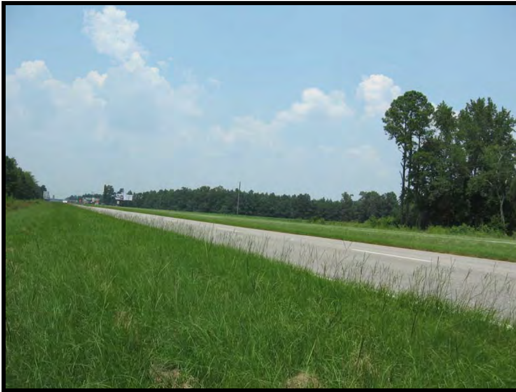
Photograph 29– Looking north along U.S. Highway 501
