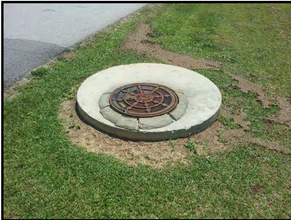
Photograph 2 – Typical manhole observed at the property
