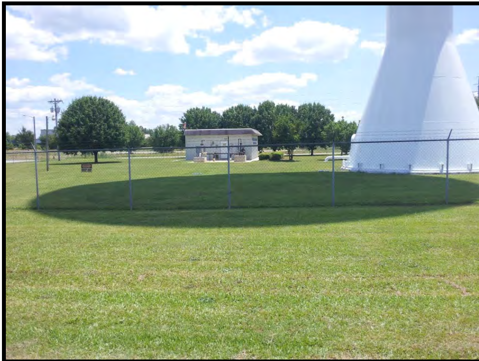
Photograph 6 – Looking south towards the Marco Rural Water Treatment plant
