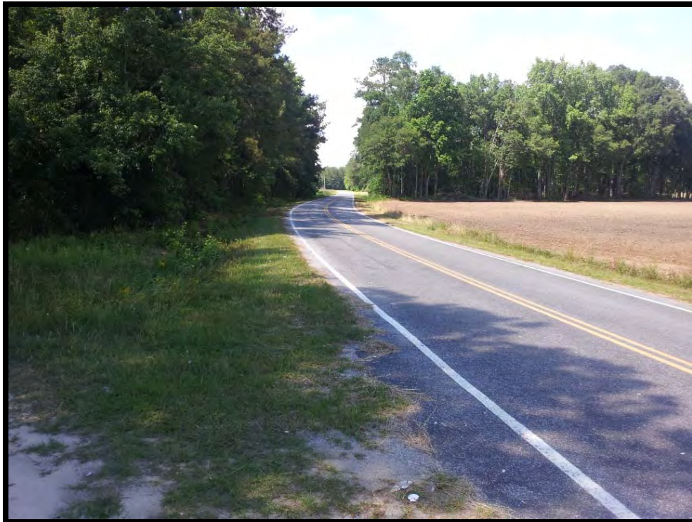
Photograph 15 – Looking northeast along Calder Road (S-34-680)
