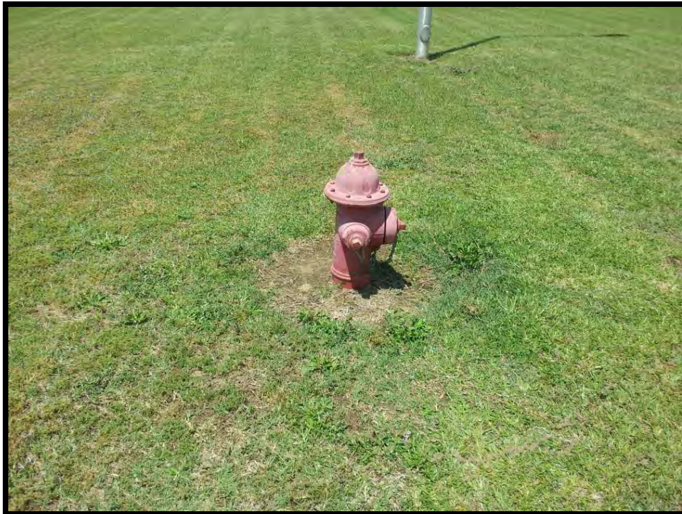
Photograph 1 – Typical fire hydrant assembly observed at the property
