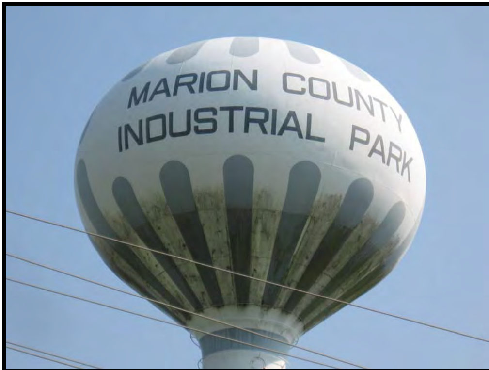
Photograph 2- Marion County Industrial Park Elevated Storage Tank
