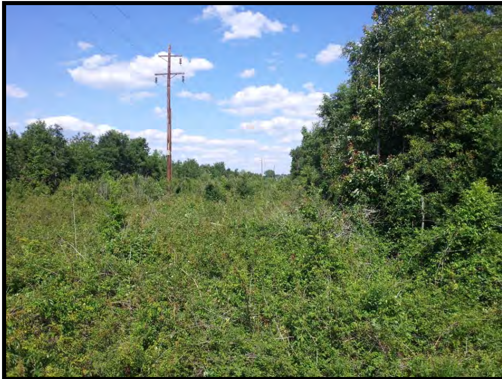
Photograph 23 – Overhead electrical power line traversing the property
