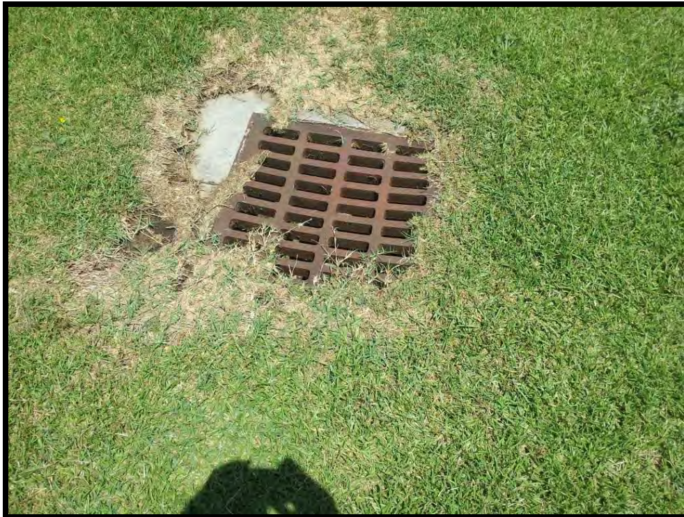
Photograph 9 – Storm drainage inlet observed on the southeastern portion of the property
