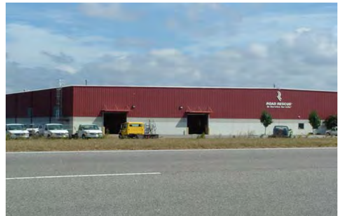
Southern adjacent property
