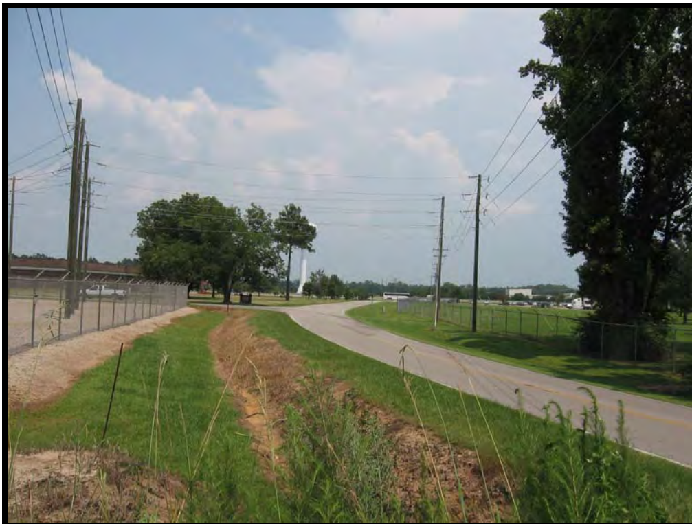
Photograph 34 – Looking east near the Pee Dee Electric Cooperative Sub-Station
