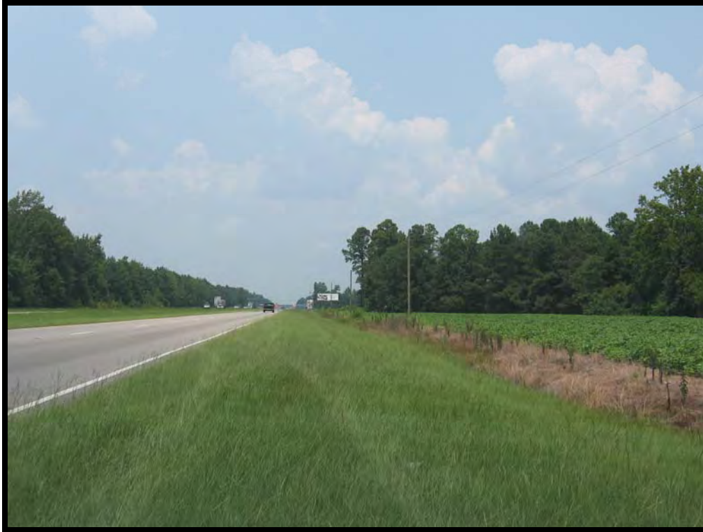
Photograph 23 – Looking north along U.S. Highway 501
