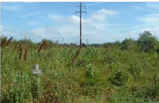
Power line crossing through middle of subject property
