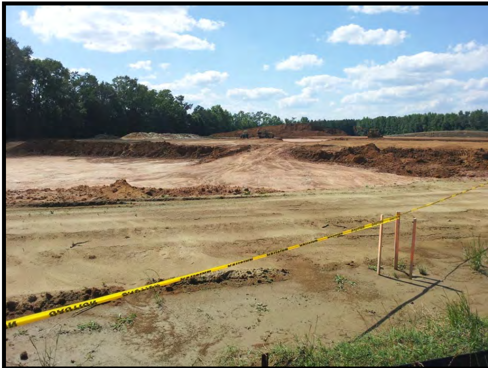
Photograph 16 – Looking north across the property towards the construction project site
