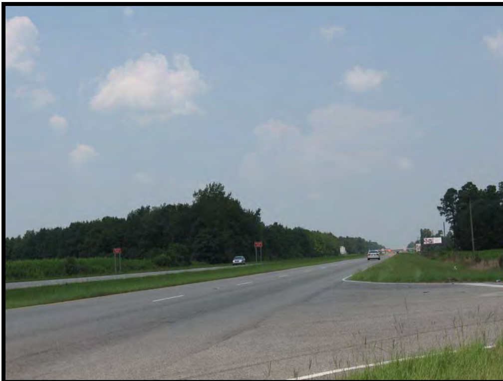
Photograph 12 – Looking north at the intersection of U.S. Highway 501 and Gurley Road
