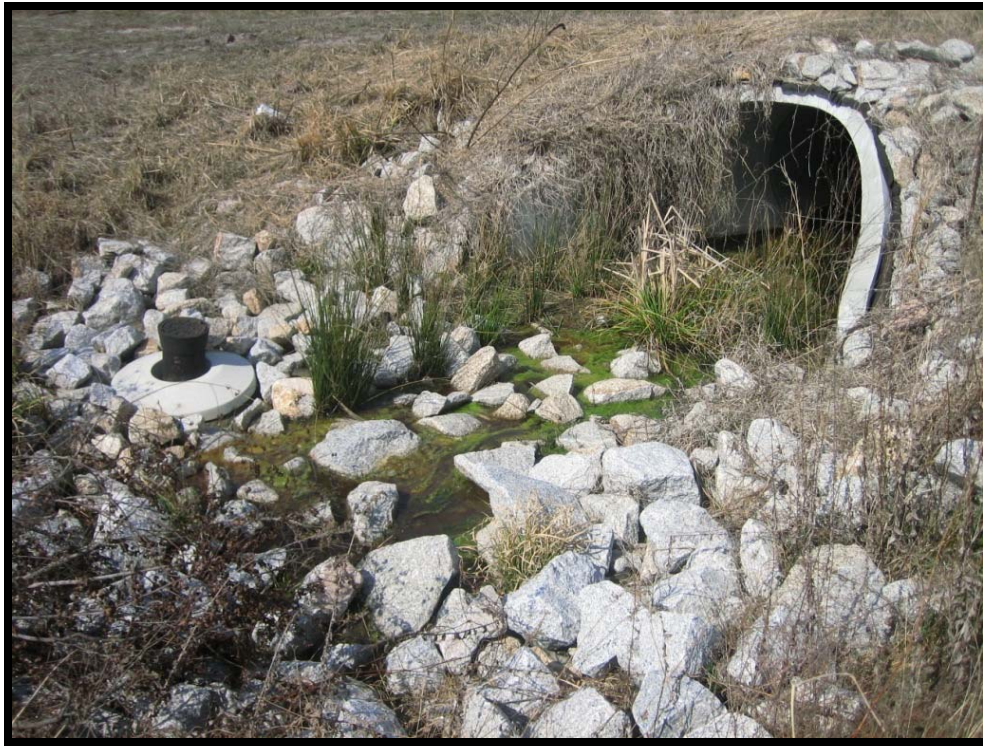
Photograph 15 – Storm drainage culvert extending beneath the roadway serving the Epps No. 1 Industrial Site
